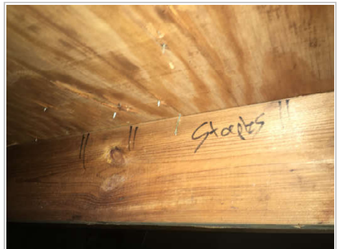
Stapled Roof Deck
